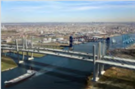
Goethals Bridge Replacement, New York, New Jersey
