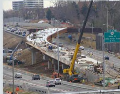
I-95 HOV/ HOT Lanes Project, Virginia
