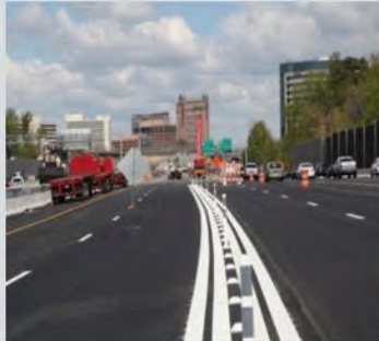
I-495 Capital Beltway HOT Lanes, Virginia
